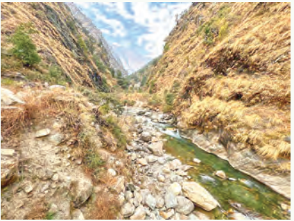
Super Ankhlu Khola Hydropower Project (25.4 MW)
