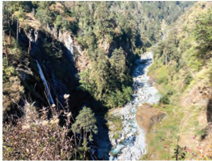
Brahmayani Hydroelectric Project (35.47 MW)
