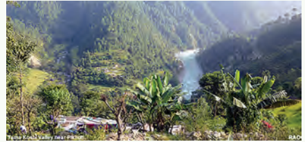
Sagu Khola 1 Hydropower Project (5.5MW)
