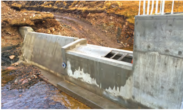
Corroul Estate Hydro Scheme_Intake (5.3 MW), UK
