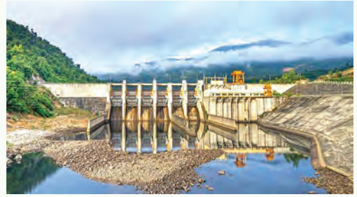
Suri Khola Hydroelectric Project (6.4 MW)
